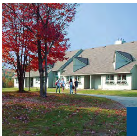
Townhouse Residence Complex 100 College Dr. North Bay, ON
