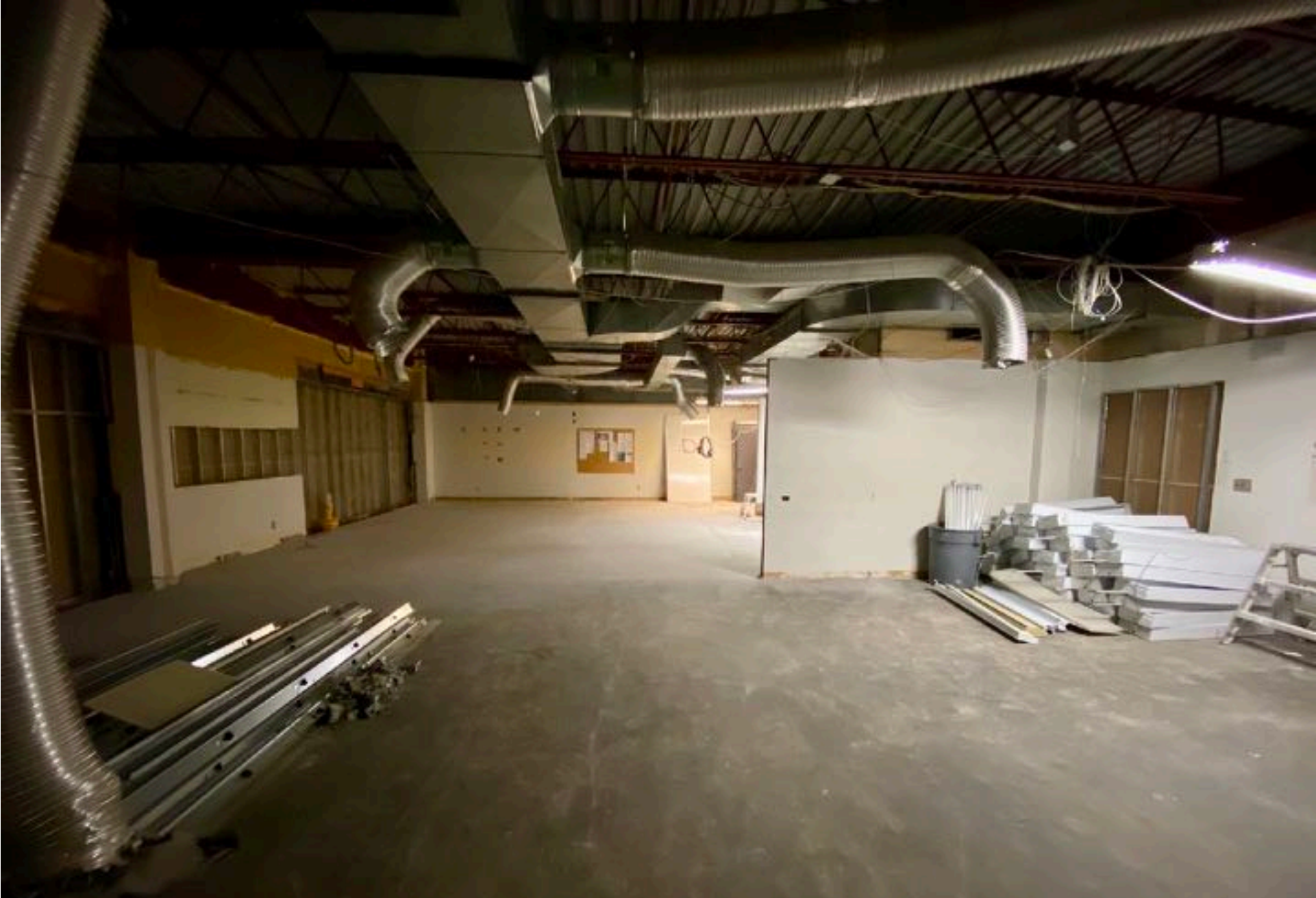
Framing Materials On-Site
