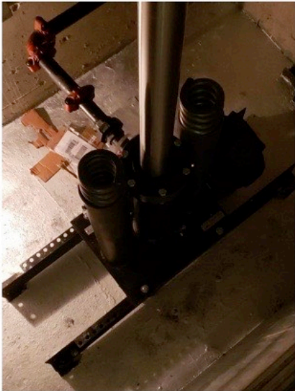
Completed Jack Unit
